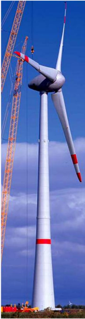
The Enercon E-126 has blades that are nearly as long as the wings of a Boeing 747 (63 meters long vs. 68 meters long). Photo from www.treehugger.com
